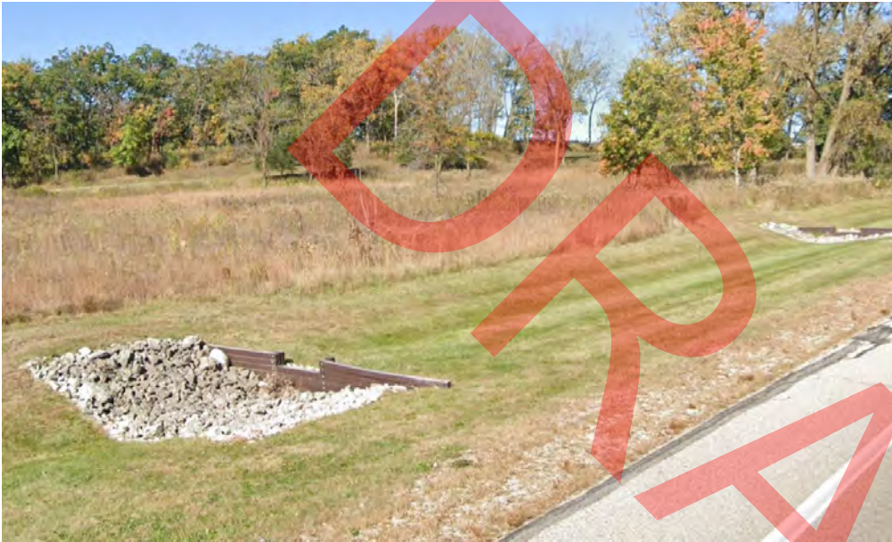
Figure 3.8 Regenerative Stormwater Conveyance Along Hwy 67
